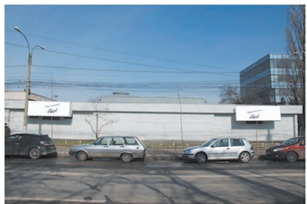
BANNER DISPLAY ON ROMEXPO HEADQUARTER FACADE
